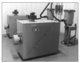
5 HP Pumps in Sound Enclosures (with dust collectors)
